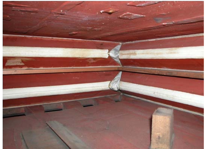
Interior of the bellows, before dismantling
