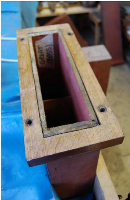
End of a wind trunk, with a loose fixing frame
