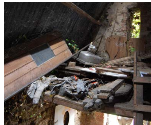
Metal pipes in the sexton's hut
