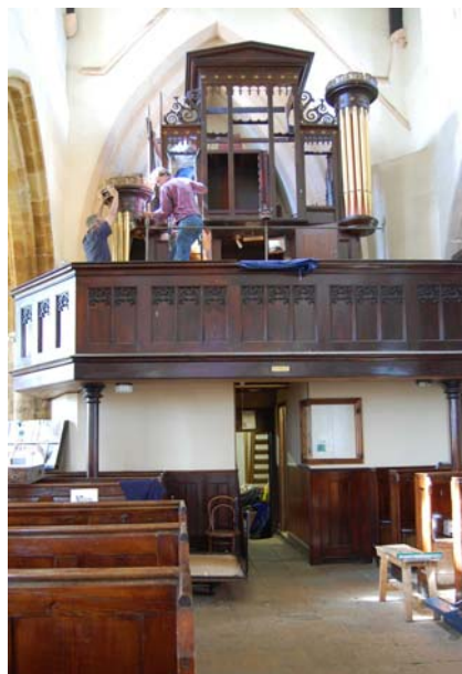
Great pipes before dismantling. Note empty holes for bottom notes and the Oboe type reed pipes.
